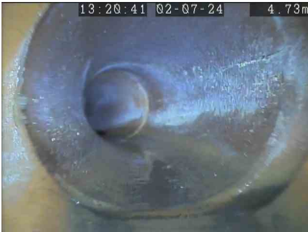
UU MH 4115X_21c7e9cd-9f85-408f-919a-1b3d42e95a3f_20240709_1 50532_358.jpg, 00:00:28, 4.73 m Open joint, medium
