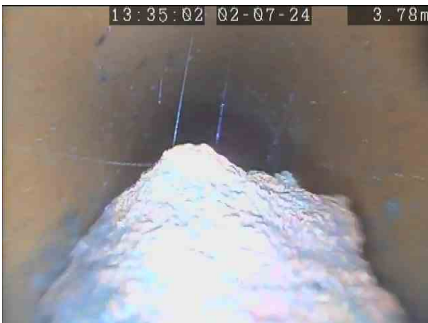
UTPX_beed247e-ce6b-4a78-a922-51fea32361c1_20240710_105441_123.jpg, 00:00:27, 3.78 m Settled deposits, other, 40% cross-sectional area loss, Debris
