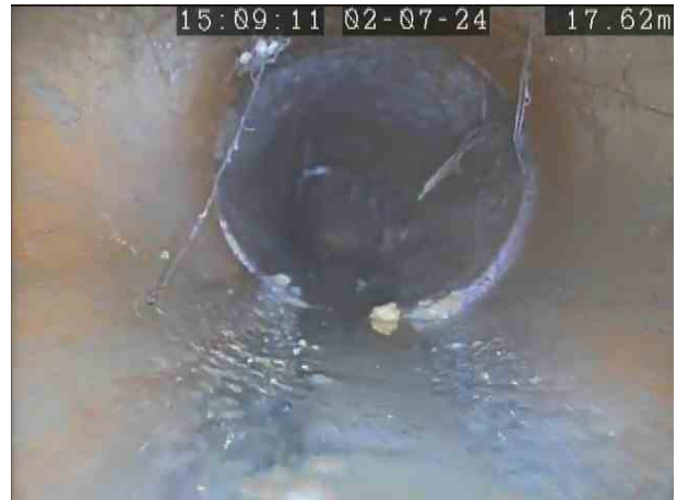
UU MH6107AX_5017909f-c386-426c-b254-316ba6b4dd71_20240 710_124341_701.jpg, 00:01:53, 17.62 m Roots, fine
