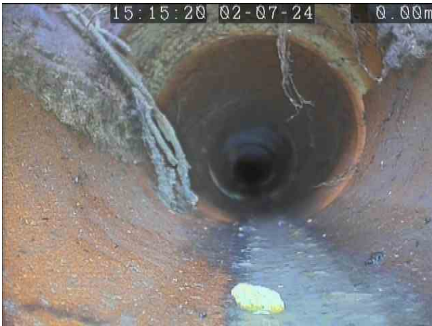
UU MH6107CX_09cbff7f-9bc6-4ce9-8915-7d9989a1bd12_202407 10_130335_944.jpg, 00:00:12, 0.01 m Roots, fine
