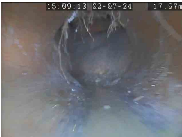
UU MH6107AX_0ec05cdd-4a87-4023-aed1-7880fe3c889f_20240 710_124400_211.jpg, 00:01:55, 17.97 m Roots, fine
