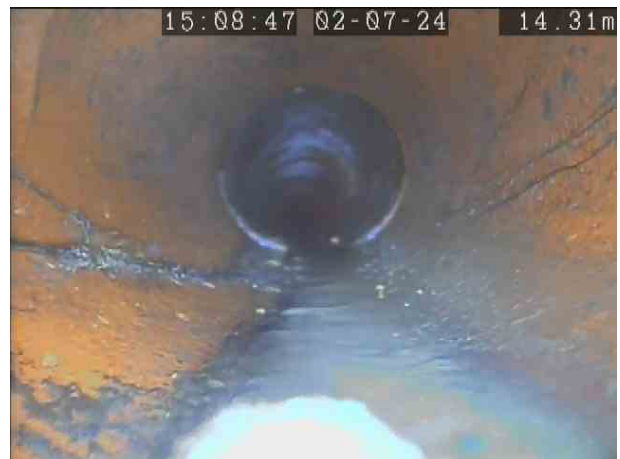
UU MH6107AX_70430c2e-8bc0-45aa-b2d9-8800030f61fd_20240710_124222_497.jpg, 00:01:29, 14.31 m Roots, fine
