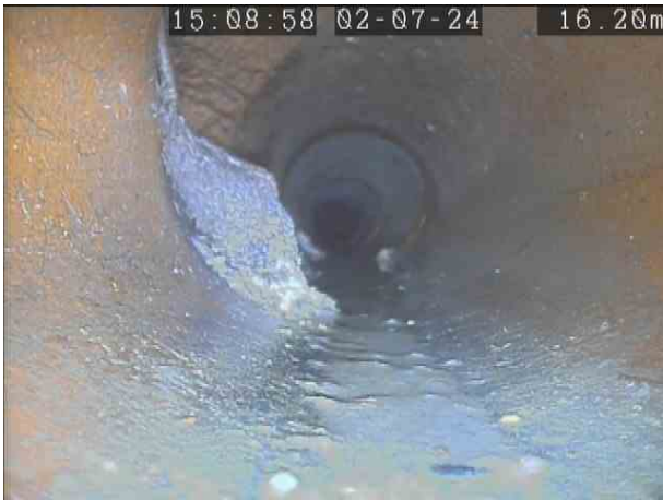
UU MH6107AX_6ede8f1f-d234-4ec7-a255-2f600592bcf3_202407 10_124318_501.jpg, 00:01:39, 16.20 m Roots, mass, 10% cross-sectional area loss
